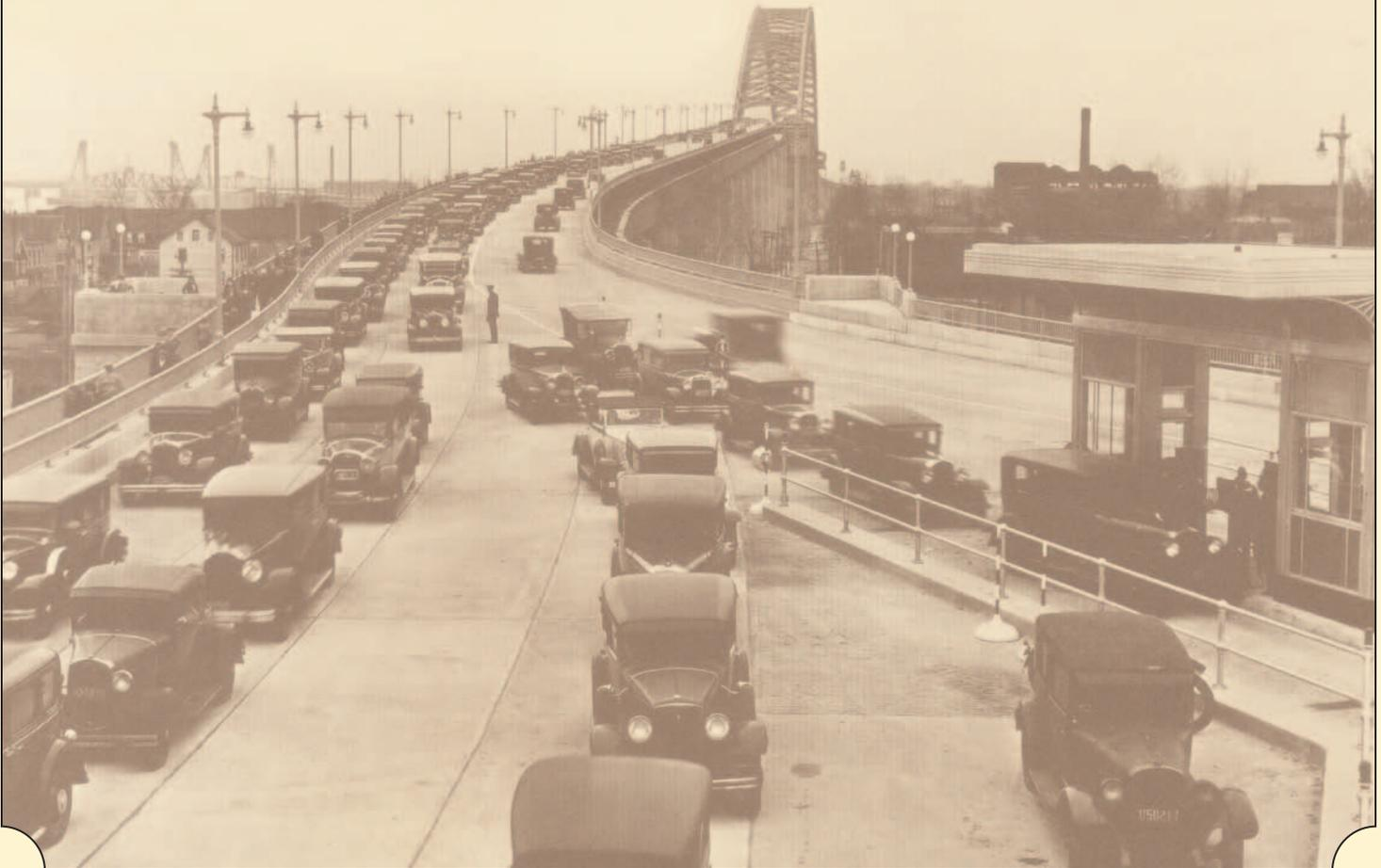
The Bayonne Bridge, with its 1,675 foot span and a clearance at the center of 150 feet, was designed to provide unobstructed passageway for the tallest ships the U.S. Navy operated. The Kill van Kull is still the main ship gateway between Newark Bay and the Hackensack and Passaic rivers to the north and the Arthur Kill to the south.
