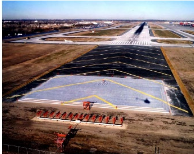
FIG 2-3-42 Engineered Materials Arresting System (EMAS)
