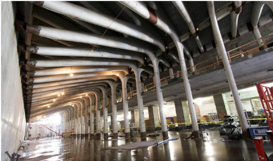
**Greenwich Street Corridor:** Soil and concrete removals, as well as rock excavation, are under way. PATH underpass slab demolition beneath the # 1 subway line is 100% complete, as is one third of structural slabs.
