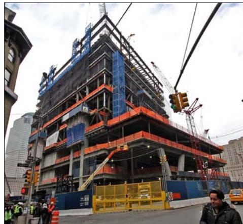
Located at the southeast corner of the site, 4 WTC will rise to 975 feet. This month, steady progress will continue on the reinforcement and form work for concrete floor slabs and columns, currently on the 5th floor. The steel erection and installation of the core wall will also continue through the 11th and 13th floors, to what will eventually be a 64-story tower.
