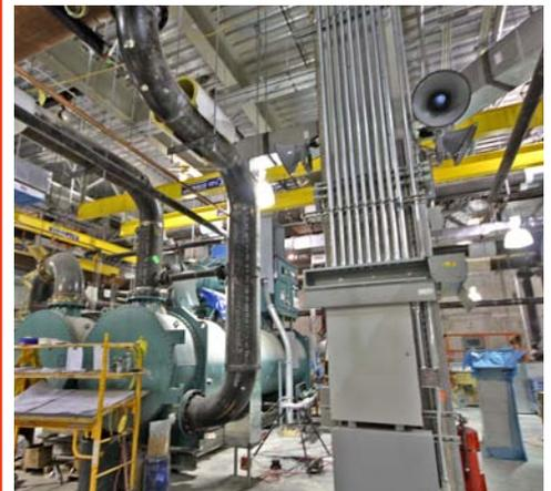
The Central Chiller Plant is a 12,500-ton capacity facility beneath the Memorial Plaza. Designed to provide air conditioning to facilities at the WTC site, it will use the River Water Pipe System to draw water in from the Hudson River through the River Water Pump House, which is currently being rehabilitated. Recent construction progress on this project includes field testing of the third 2,500 ton chiller for leaks and the delivery and rigging of the 40 volt switchboard.
