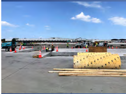
Slab Removal / Replacement at Taxiway UA
