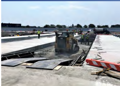
Concrete Slab Replacement at Taxiway UA
