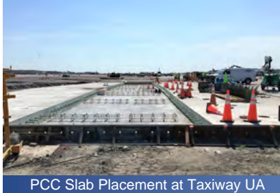
PCC Slab Placement at Taxiway UA
