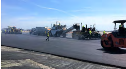
Asphalt Placement at Taxiway U
