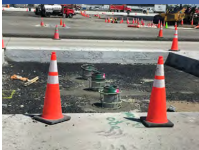
Typical Light Can Installation
