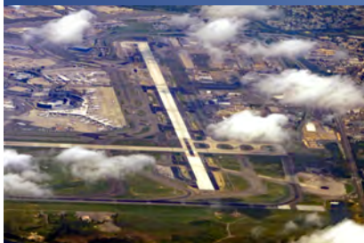
Construction Progress - Aerial Photo
