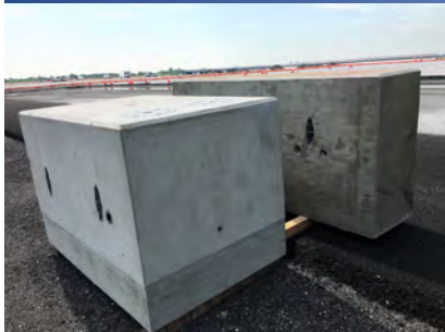
Foundations for FAA PAPI System
