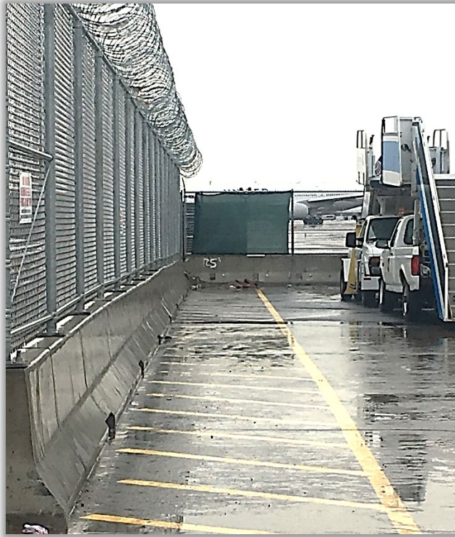
Figure 7 – Example of Port Authority AOA Security Fences
