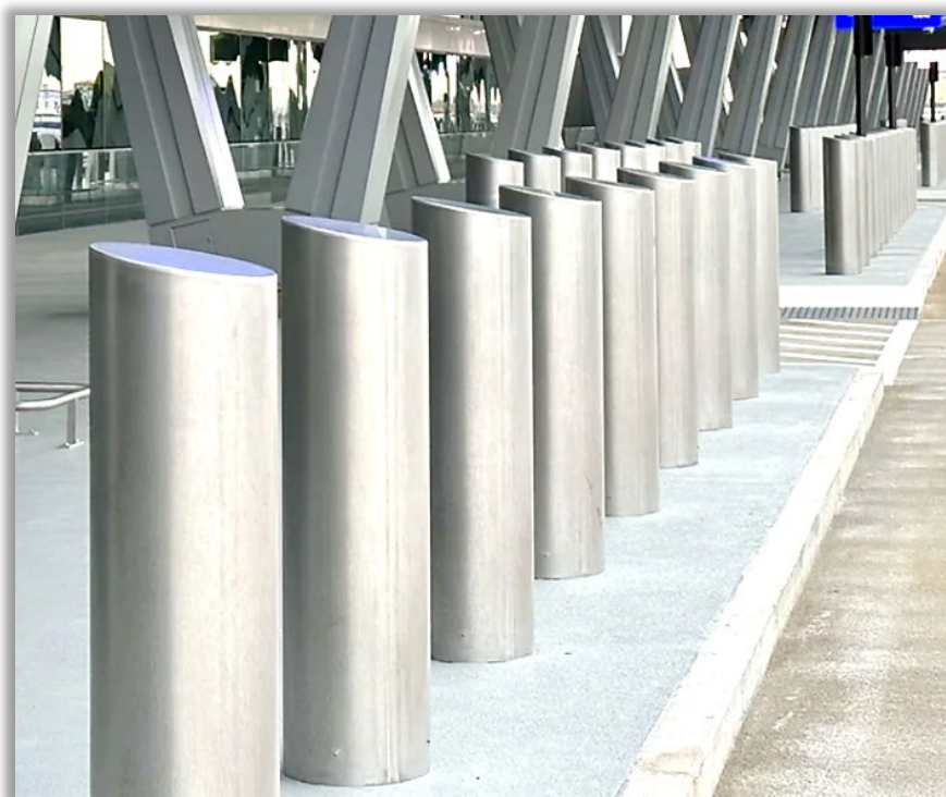
Figure 2a – Security Bollards at Terminal Frontage Roadway
