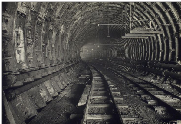
Inside the Holland Tunnel during construction.
