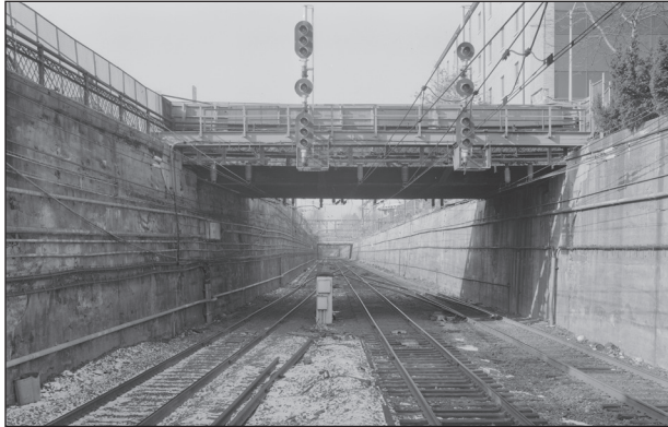
Left: Beam bridge spanning New Jersey Transit Tracks. Maple Street Bridge, Summit, New Jersey.
