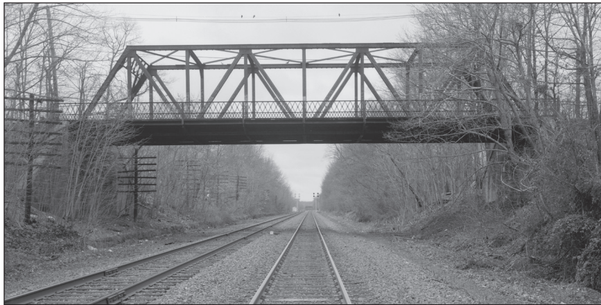
Right: Old Stone Bridge, Boonton, New Jersey.
