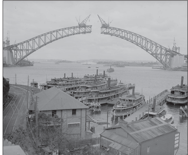
Sydney Harbour Bridge, Sydney Australia, during construction.
