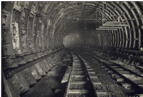
Inside the Holland Tunnel during construction.
