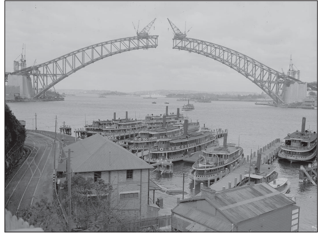
Sydney Harbour Bridge, Sydney Australia, during construction.
