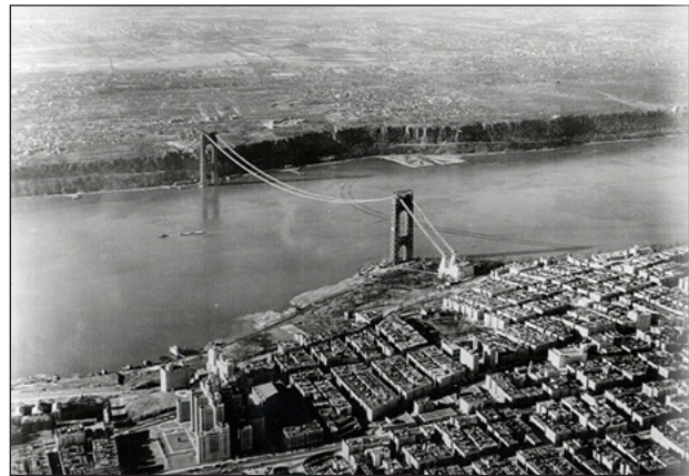
George Washington Bridge during construction, before the roadway was built.
