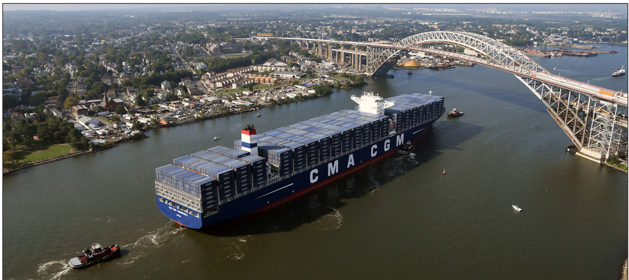
A New Panamax Ship passes under the Bayonne Bridge in 2017 after the roadway was raised.
