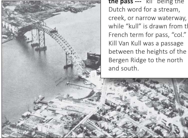
Aerial view of the Bayonne Bridge during construction.
