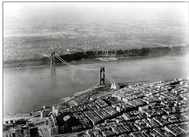
George Washington Bridge during construction, before the roadway was built.
