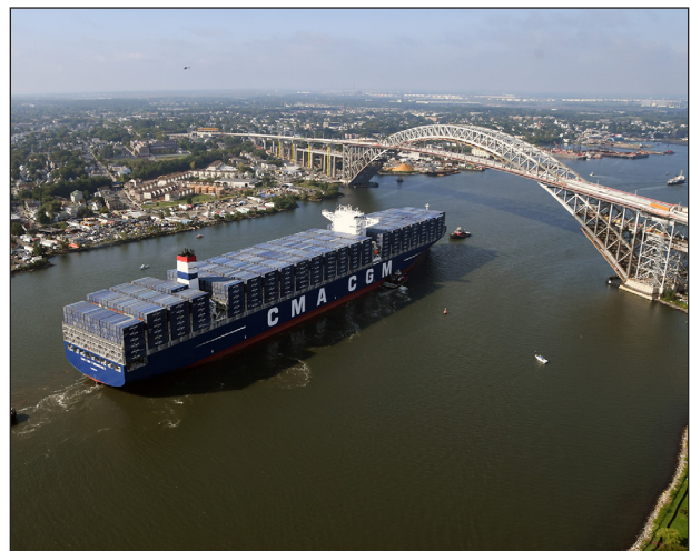
A New Panamax Ship passes under the Bayonne Bridge in 2017 after the roadway was raised.
