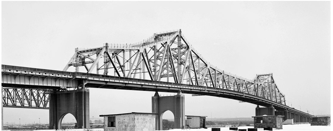
Goethals Bridge as it exists today (Joseph Elliott 2014)
