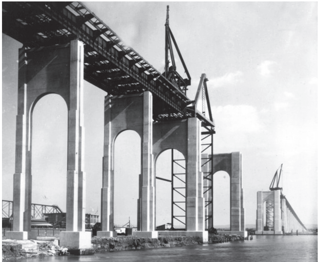
Goethals Bridge under construction, 1926 (Courtesy of PANYNJ)
