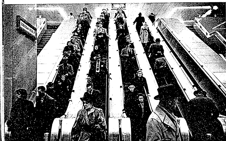
This bank of five motor stairs carries passengers between the main concourse and the suburban level. There are 31 motor stairs in the terminal.
