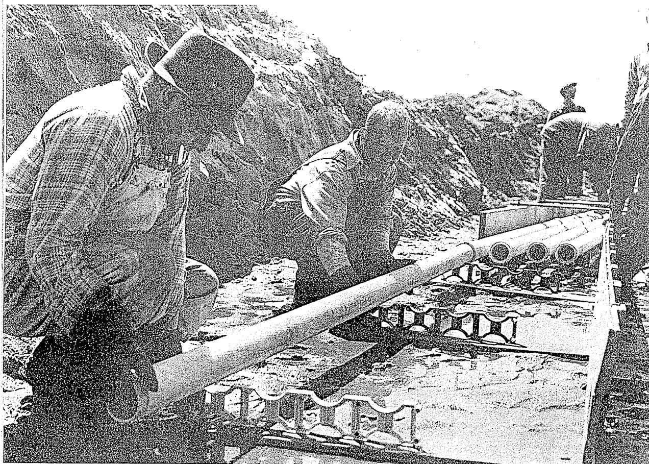
At International Airport asbestos-type duct is installed to house electrical cable for the temporary fuel storage facility which was enlarged during 1951 to a capacity of 1,020,000 gallons.
