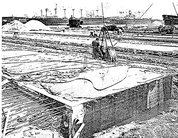
Concrete foundation is laid for Port Newark transit shed.
