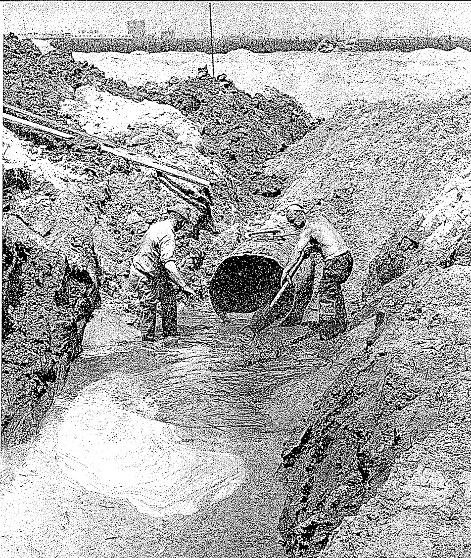
Workmen excavate ahead of this 36-inch culvert pipe, part of extensive drainage system necessary for construction of new 7,000-foot Runway A and adjoining taxiways at Newark Airport.
