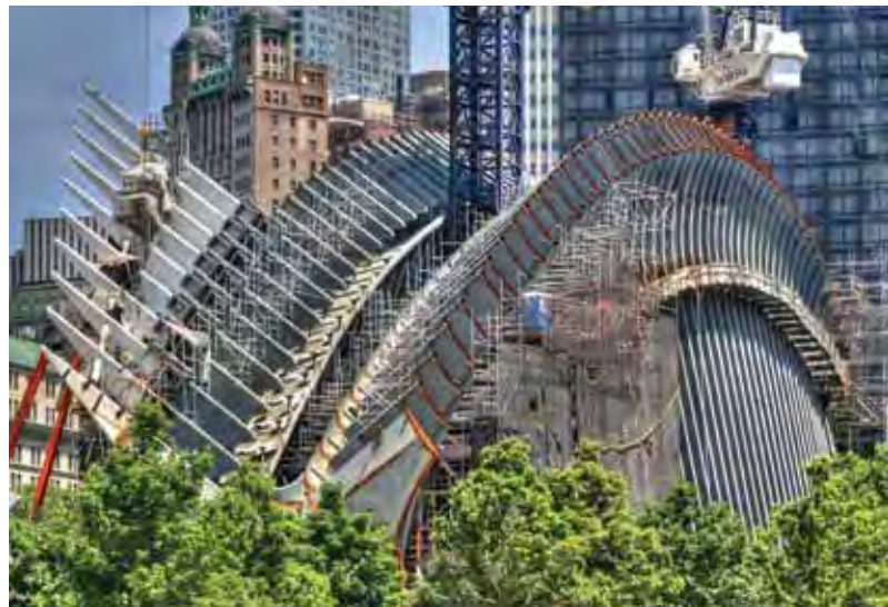
On a daily basis, the WTC's Transportation Hub will connect some 200,000 commuters with the most integrated network of underground pedestrian connections in New York City.
