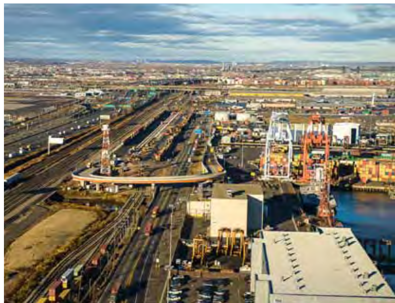
A new flyover at Port Newark smooths the flow of truck and rail traffic along Corbin Street.
