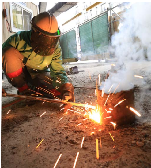
Redevelopment of the George Washington Bridge Bus Station began in August 2014. The project is expected to generate $31.7 million in total regional economic activity.
