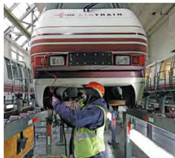
The new AirTrain Newark will offer enhanced capacity, better service, and increased reliability for area commuters.
