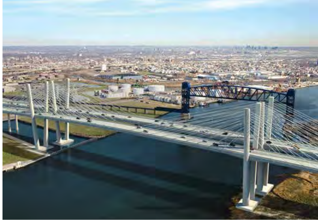
The Goethals Bridge Replacement Project is a $1.5 billion public-private partnership.
