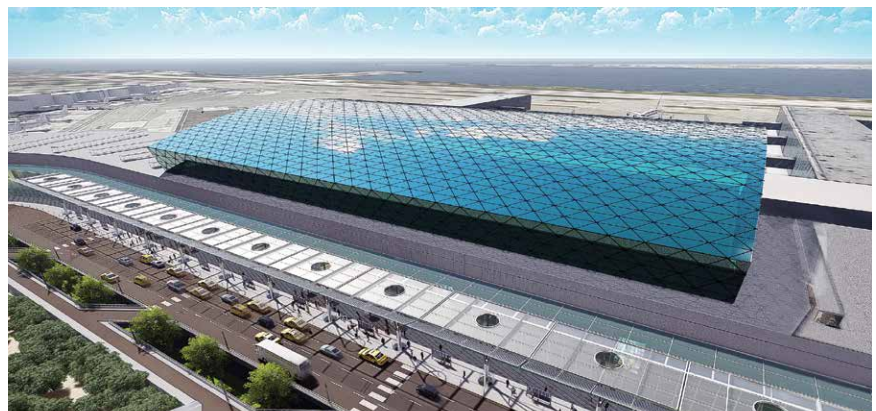
Investments for John F. Kennedy International Airport, as depicted in this rendering, will help serve the region's growing population.
