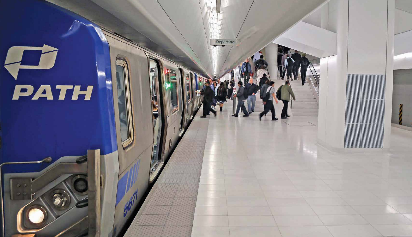
The state-of-the-art World Trade Center Transportation Hub, completed in 2016, serves 250,000 PATH daily commuters and millions of annual visitors from around the world.
