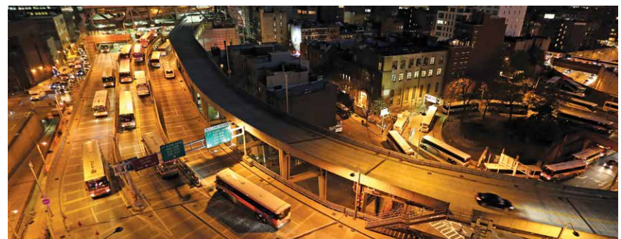
Replacing the bus ramps and slabs is essential to maintaining the current Port Authority Bus Terminal in a safe and effective operational state.
