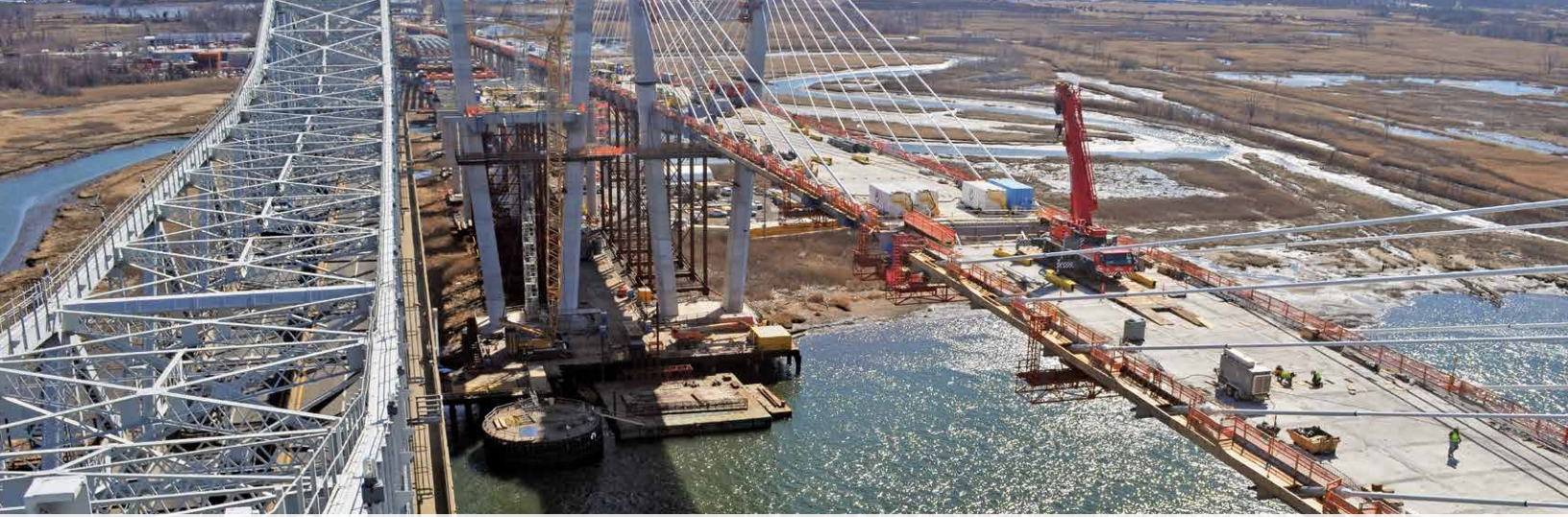
Construction proceeds on the new Goethals Bridge.
