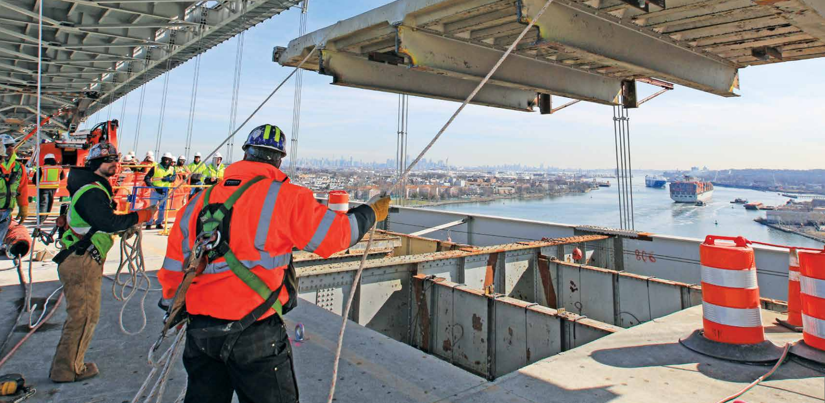
Once the newly elevated Bayonne Bridge opened to drivers, the project's work shifted to removing the old roadbed, thereby offering the proper clearance for larger neo-Panamax vessels.
