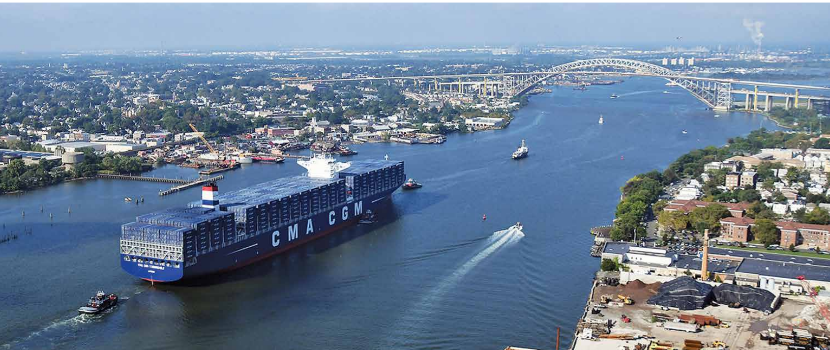
Bayonne Bridge achieved navigational clearance of 215 feet allowing larger cargo vessels to call the Port of New York and New Jersey.
