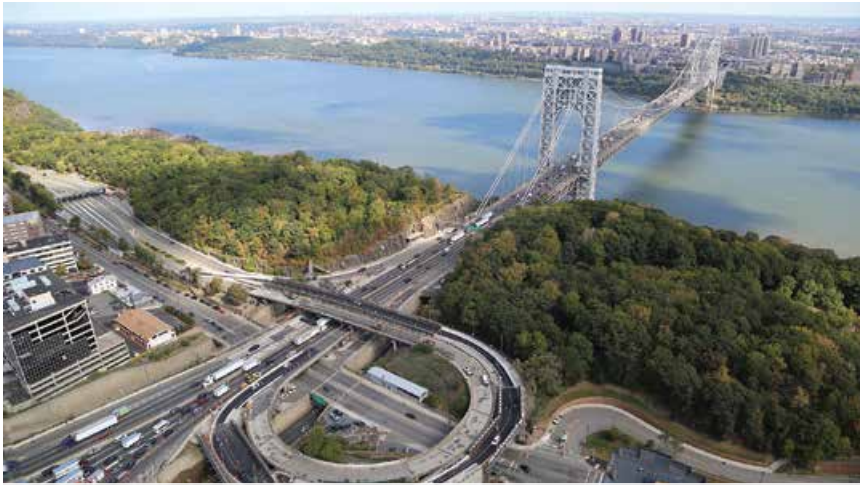
Approaches leading to the George Washington Bridge.
