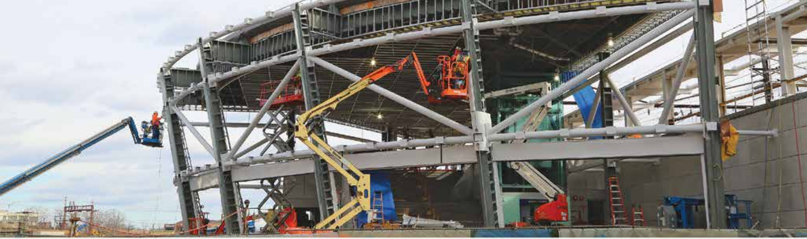
Construction continues at the new PATH Harrison Station.
