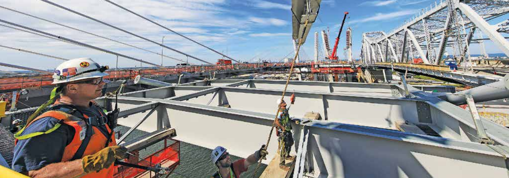
Construction progresses on the Goethals Bridge Replacement.
