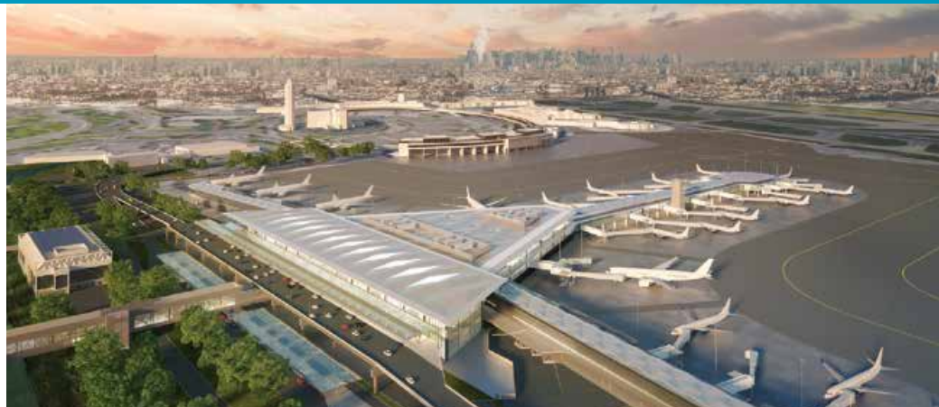
The future Newark Liberty International Airport Terminal One.
