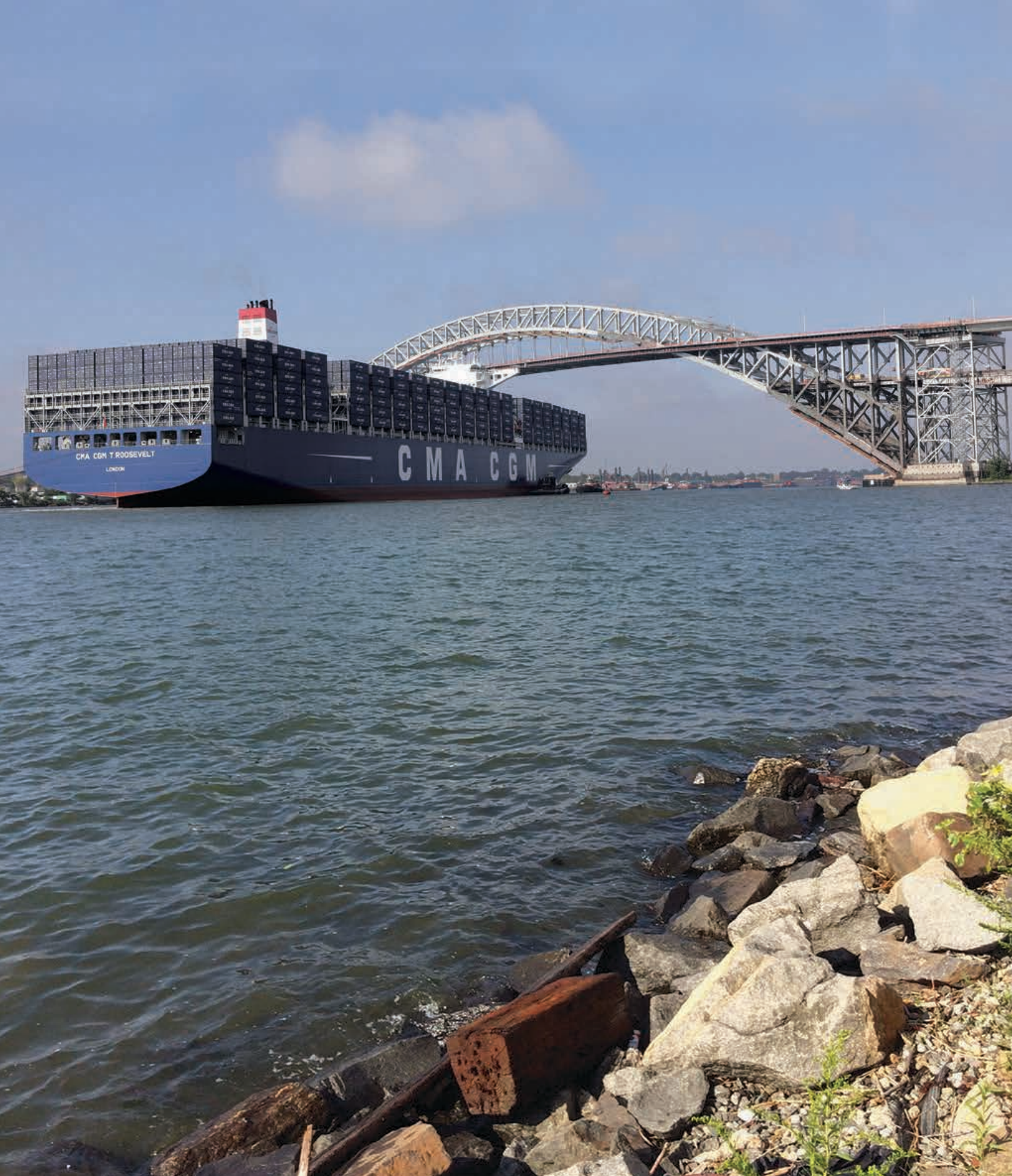
The CMA CGM T. Roosevelt approaches the Bayonne Bridge, whose new span has been elevated from 151 feet to 215 feet, enabling the newest class of container ships to pass beneath en route to Port of New York and New Jersey.
