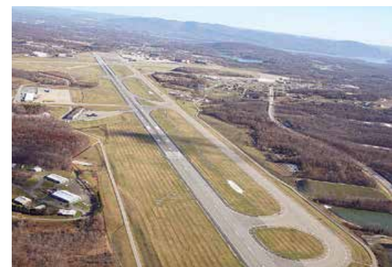
Aerial photo of Stewart International Airport.
