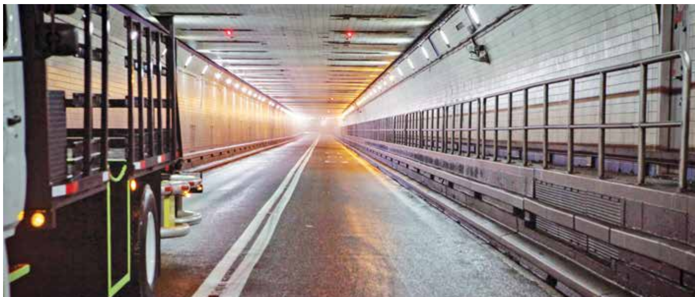
New LED lighting installation at the Lincoln Tunnel.
