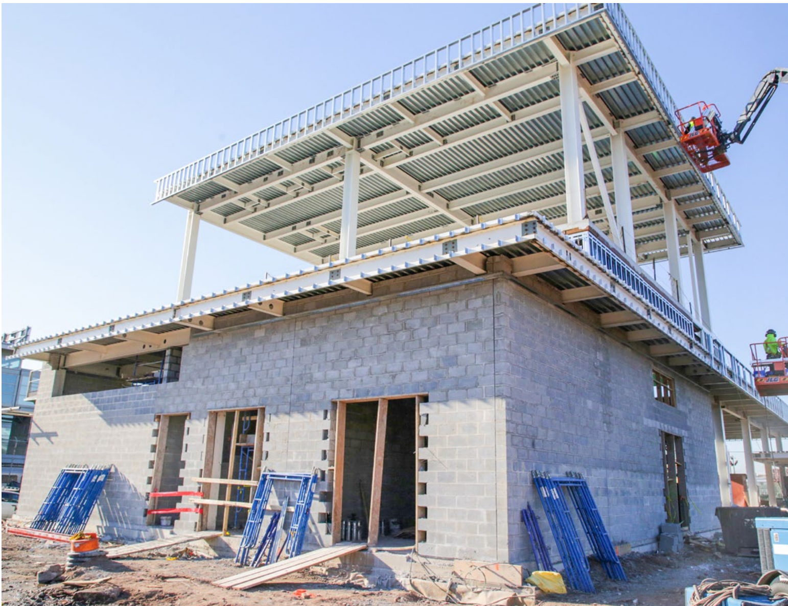
Construction of the new access point at the Newark Liberty International Airport Rail Station.
