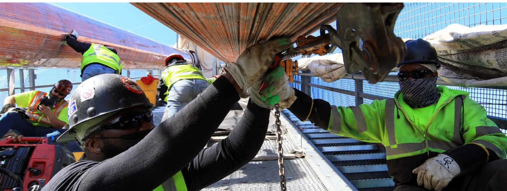
Work crews replacing steel suspender ropes at the George Washington Bridge as part of the Restoring the George program.
