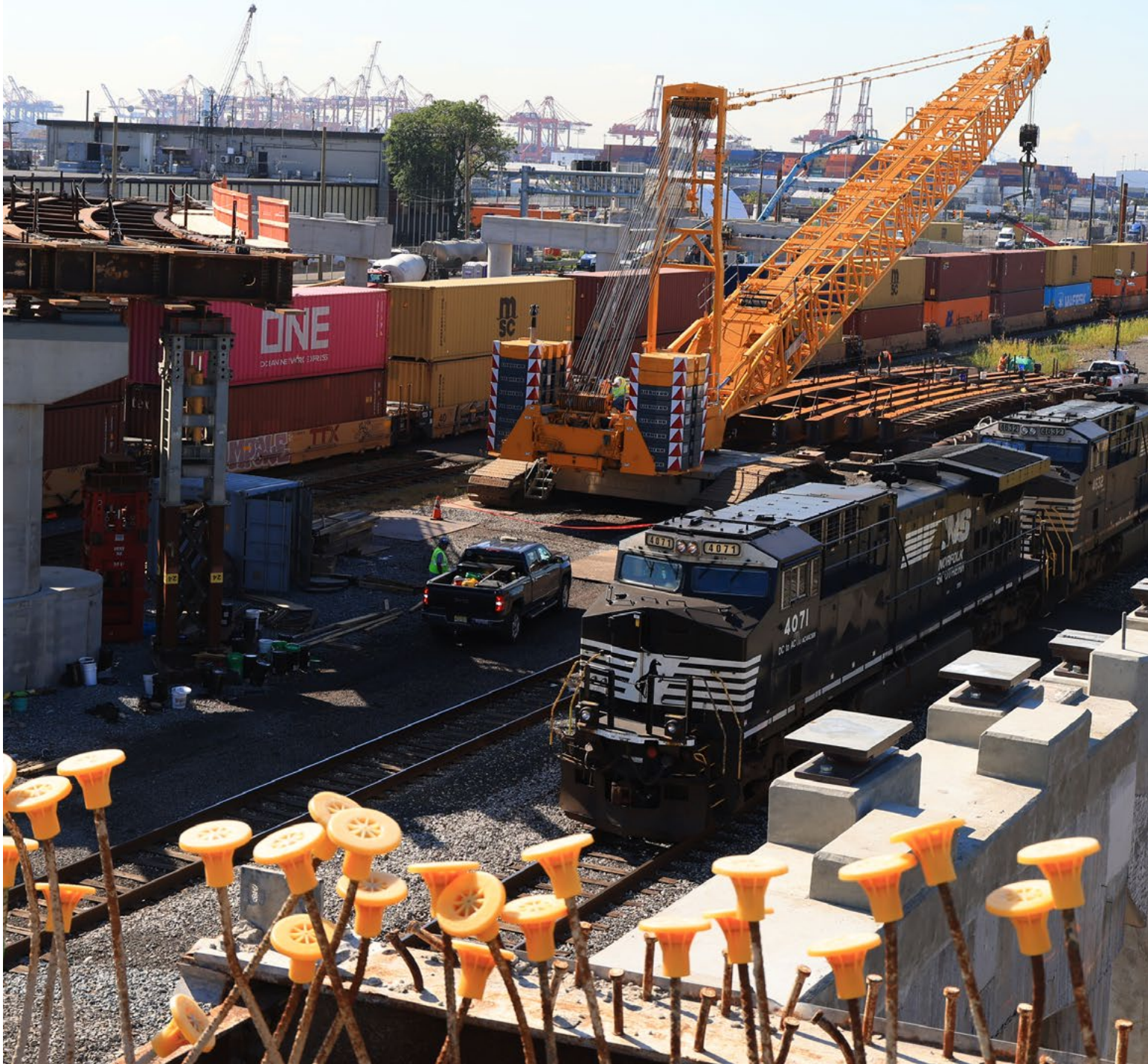
Construction progresses on the Corbin Street ramp, a pivotal phase of the Port Street Corridor Improvement Project at the Port of New York and New Jersey.
