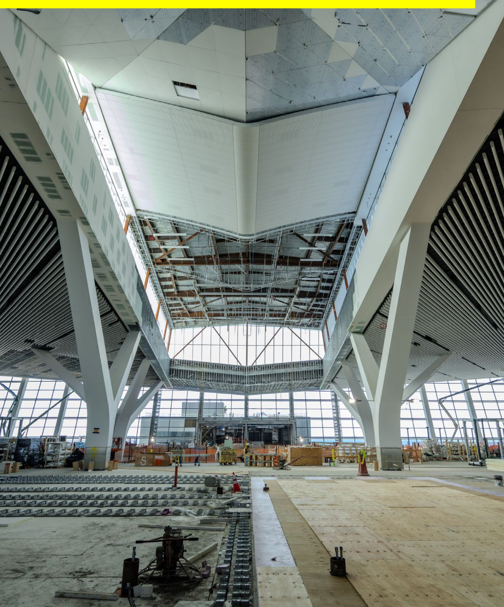
Construction progresses on the expansive departures hall at John F. Kennedy International Airport's New Terminal One.
