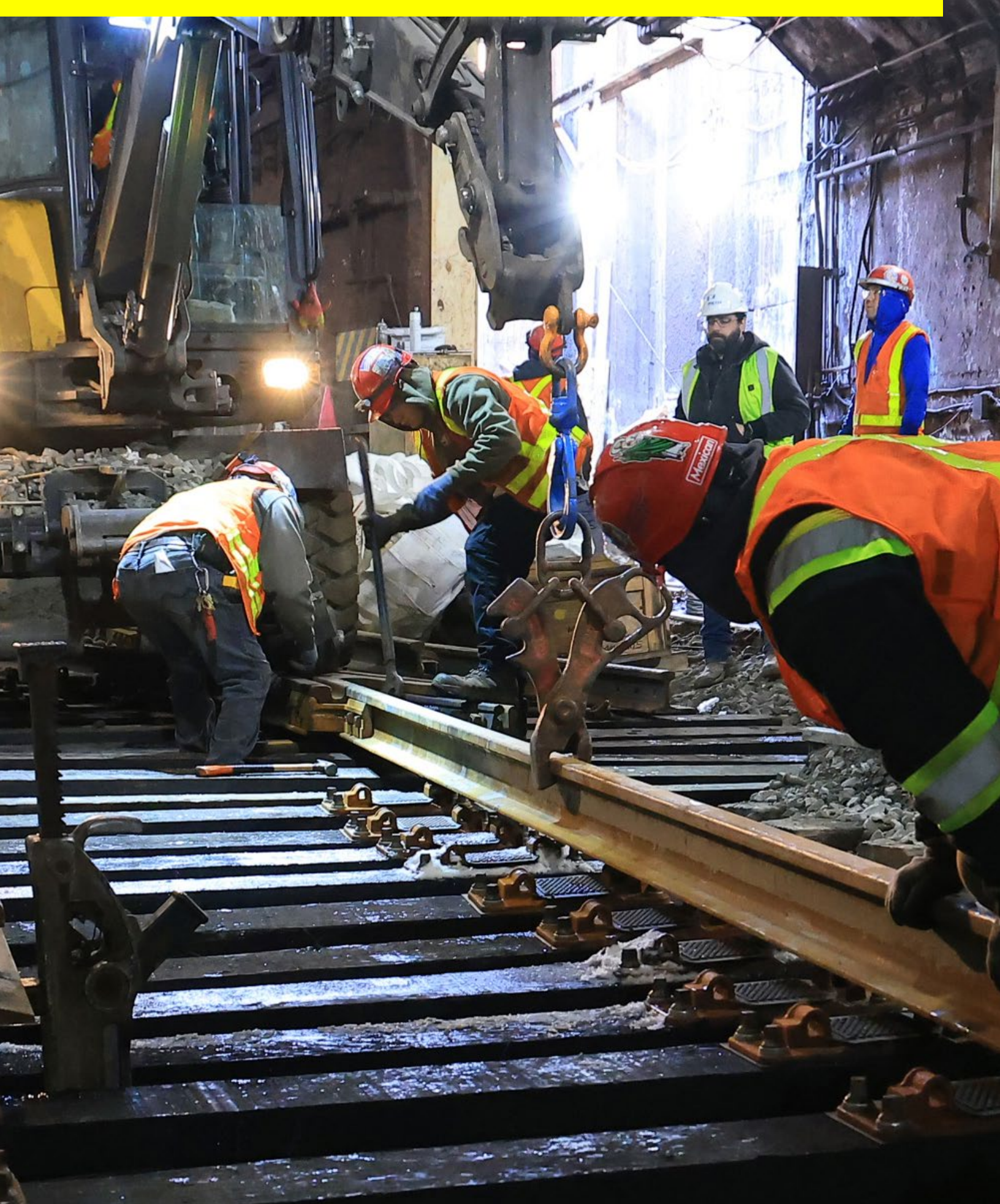
Critical track replacement during the 25-day closure under the PATH Forward Modernization Program.
