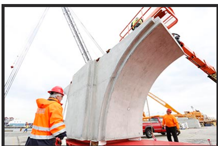
An 84-Ton Pier Capital Segment for the Bayonne
