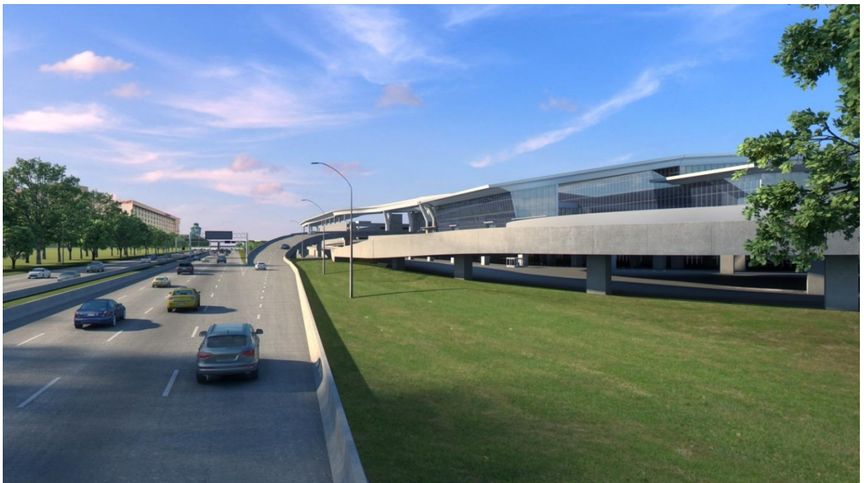
Figure 5-10. View from Grand Central Parkway (Westbound) with Proposed Action
