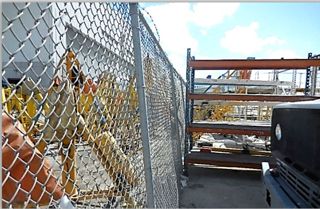
Figure 8 – Example of AOA Clear Zone Violation by Stored Objects
