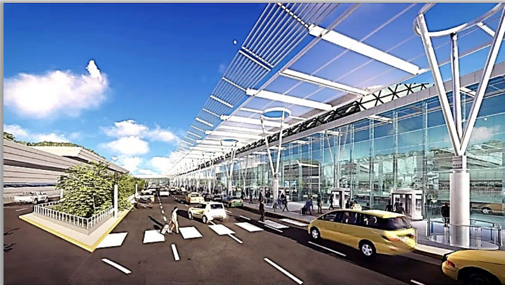
Figure 3 – Blast Resistant Cable Supported Building Facade
