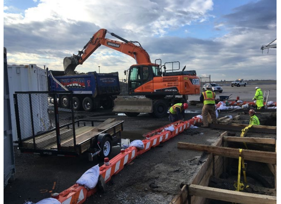
Utility Work at JFK International Airport
