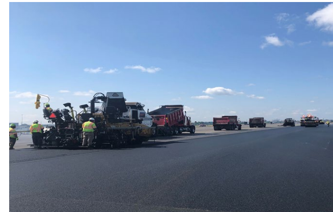
Newark Liberty International Airport Runway 4R-22L
