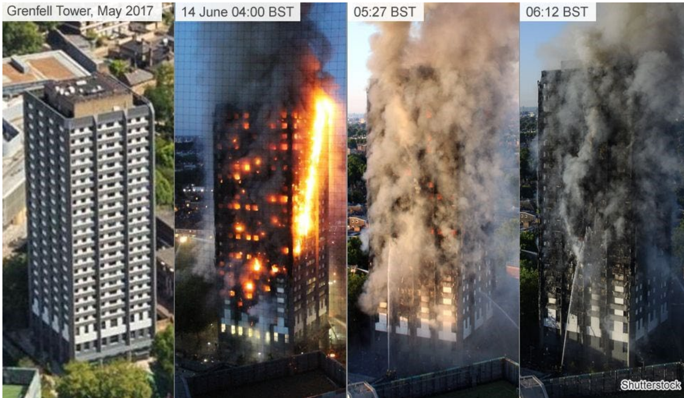
'Chimney effect' of exterior cladding
