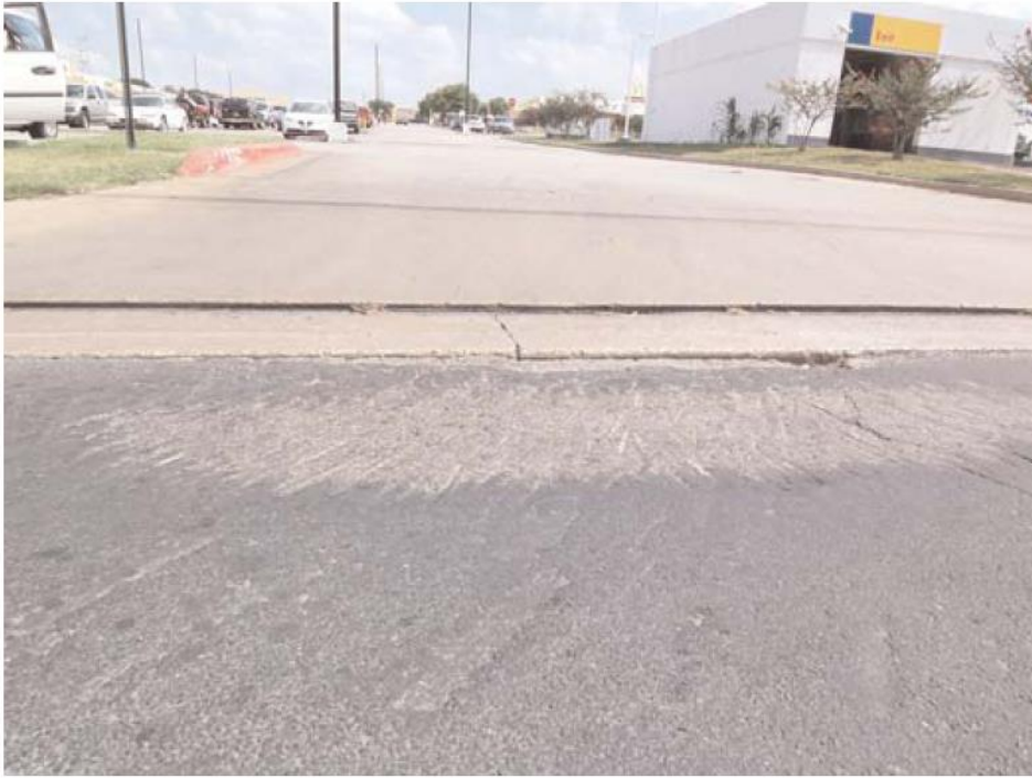
Photo 9-2: Undercarriage Scraping at Driveway due to Inadequate Vertical Profile
