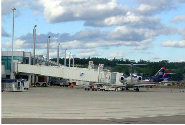
Figure 19: Passenger Boarding Bridges
