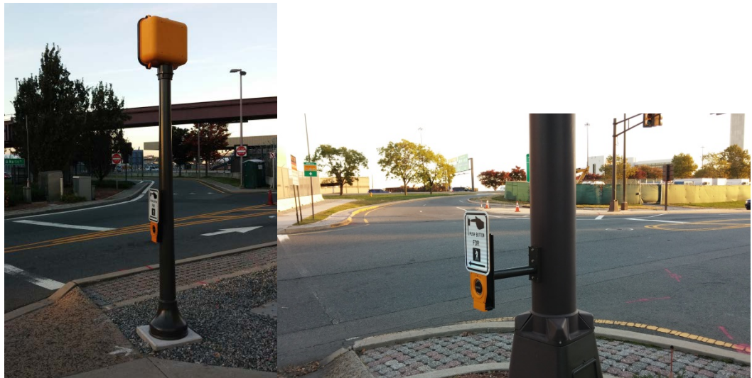
Figure 1: Proper Push Button Orientation
