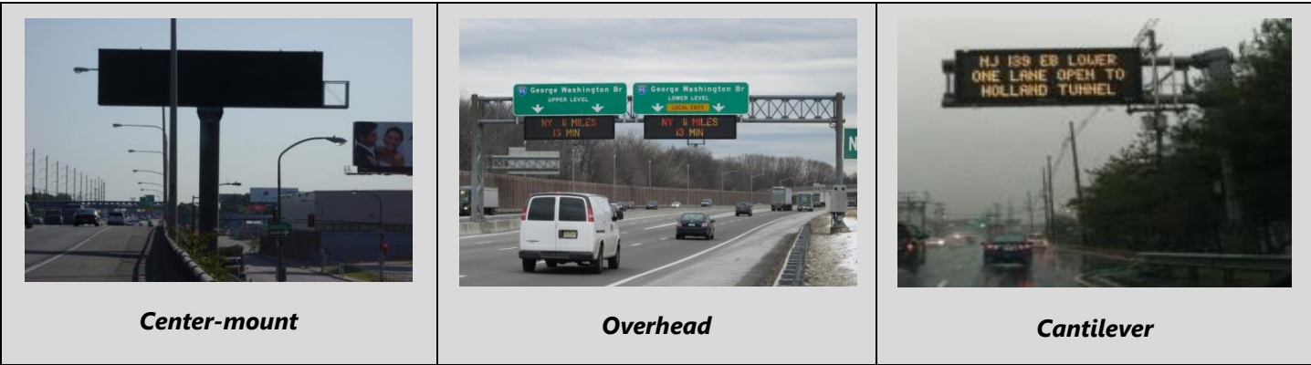
Figure 4-9: DMS Structure Types
