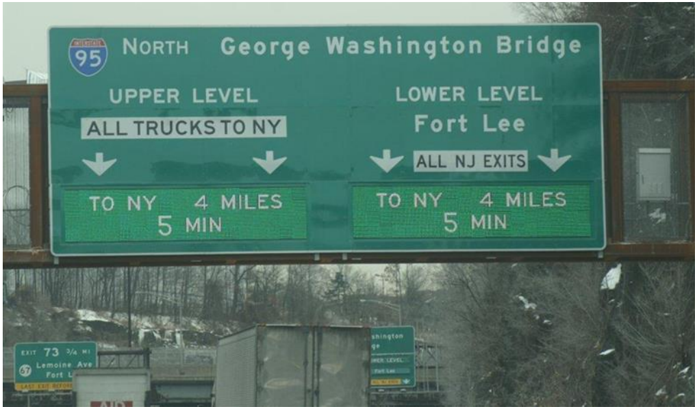
Figure 6-8: Travel Time Display on a DMS
