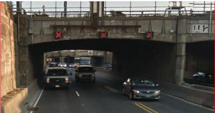
Figure 5-3: LUCS on Existing Structure
