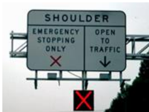
Figure 5-4: Regulatory Combined with a Lane Use Control Signal. Photo Credit: VDOT
