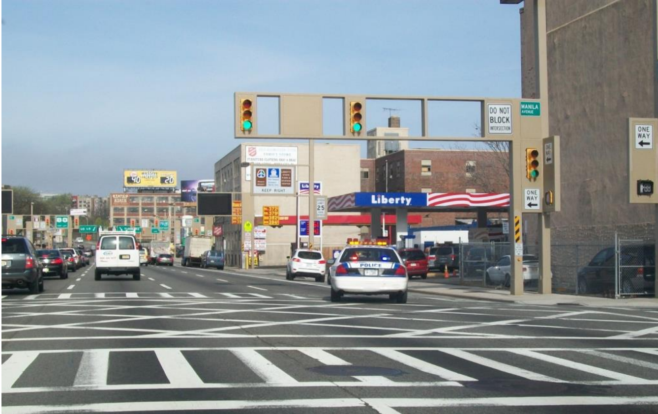
Photo 7-1: “Do Not Block Intersection” Sign and Cross-Hatched Striping at Intersection
