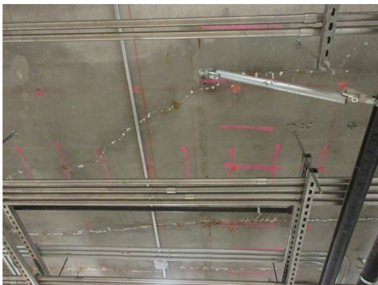
Figure 5. Representative condition of cracks in elevated slabs (underside)
