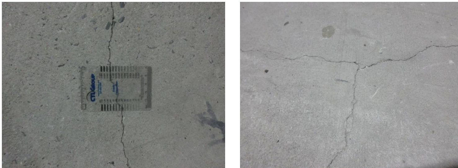
Figure 4. Representative condition of cracks in elevated slabs
