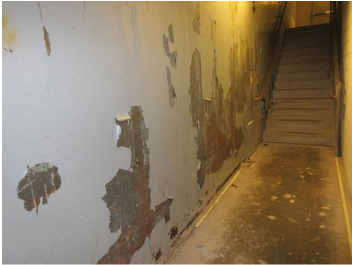
Figure 2. Representative condition of steel plates (walls) in CFP
