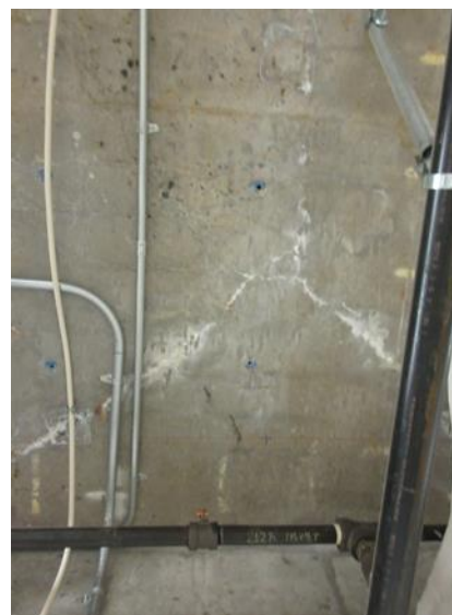
Figure 5. Representative condition of cracks in elevated slabs (underside)
