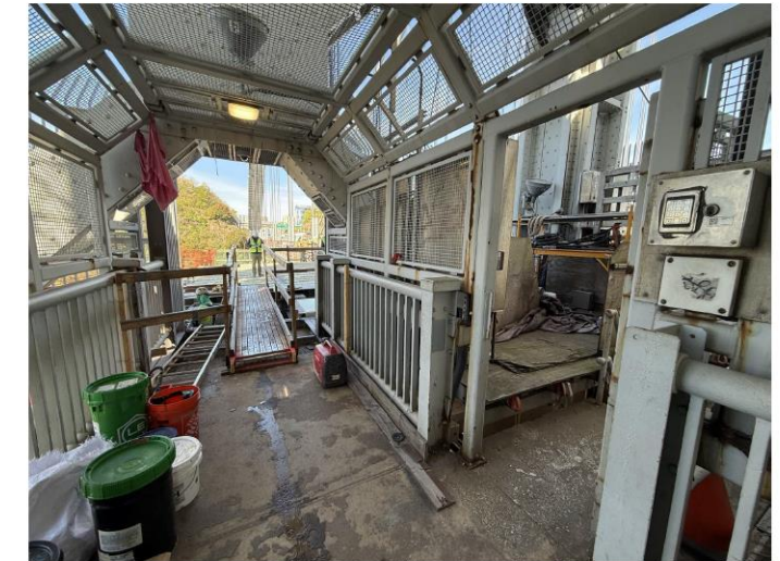
2 TOWER AREA SIDEWALK AND ENTRANCE TO UPPER LEVEL PLATFORM AREA LOOKING WEST
