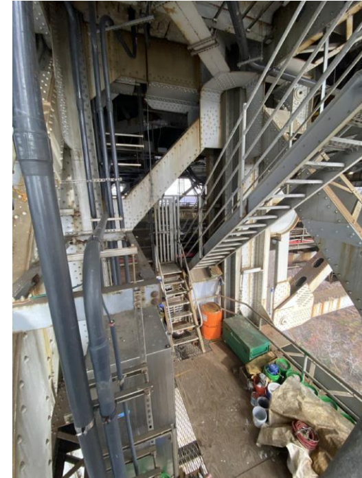
NY Tower Lower Level Platform and Stairway from Upper Level
