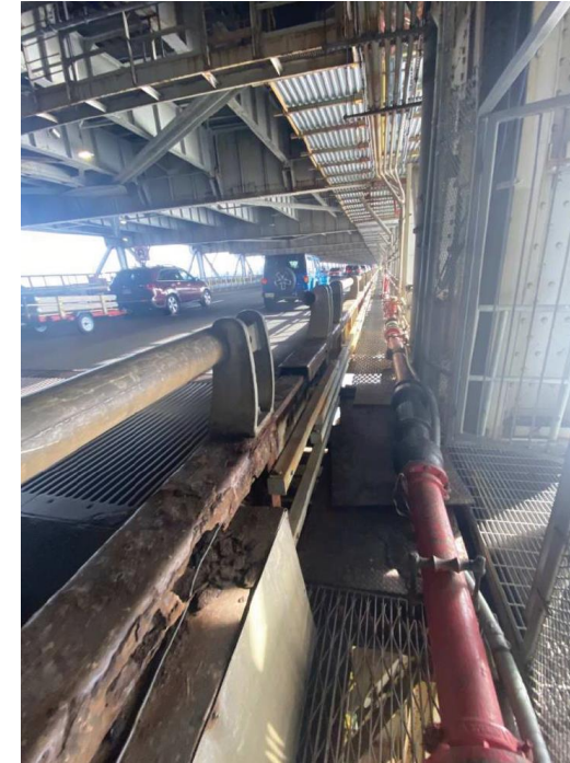
Maintenance Catwalk and Entrance to NJ Lower Level Platform
