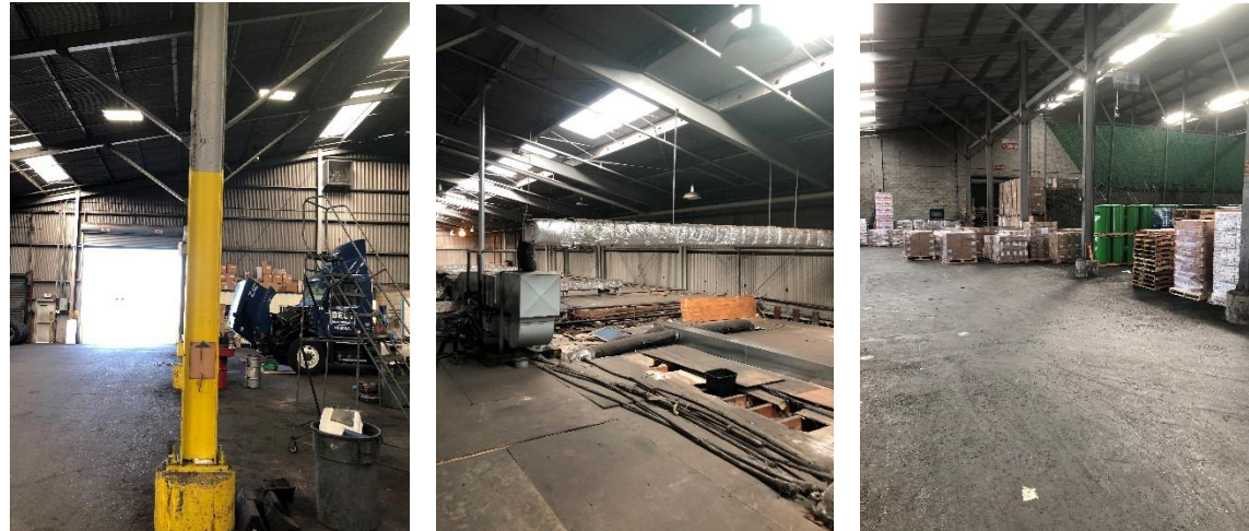
Architecture Fig 05-07 – West Side Warehouse, Partial Mezzanine, West Side Warehouse
