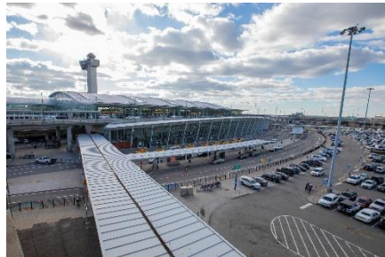
Aerial view of Blue Lot & Terminal 4
