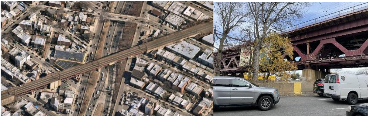
FIGURE 3.2-3: OVERHEAD VIEW AND VIEW FROM ASTORIA BLVD SOUTH LOOKING NORTHEAST OF THE HELL GATE RAIL TRESTLE
