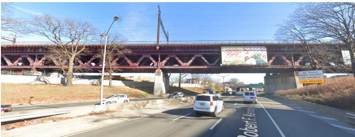
FIGURE 3.2-4: VIEW OF THE HELL GATE RAIL TRESTLE FROM THE GCP LOOKING EAST
