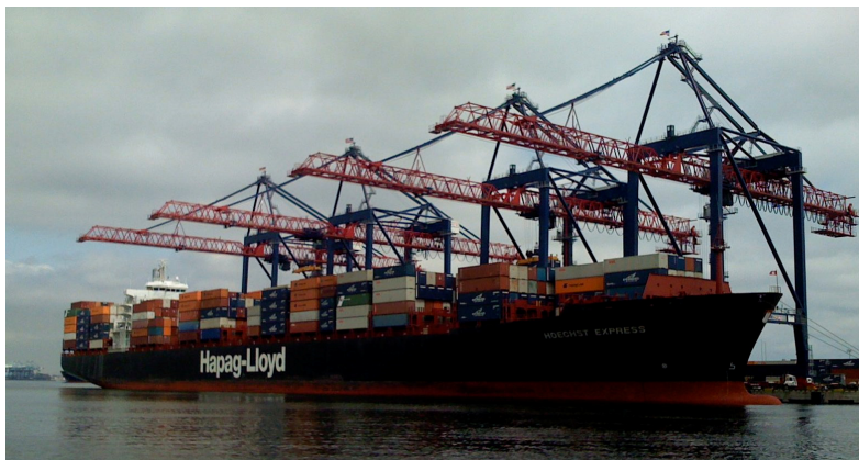
Figure 5.6: Containership at Berth
