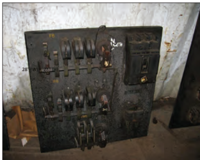
North Side Speed Control with Circuit Breaker Board
