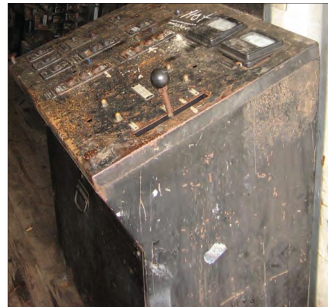
Operator's Control Stand, Bridge Motors and Winch Control
