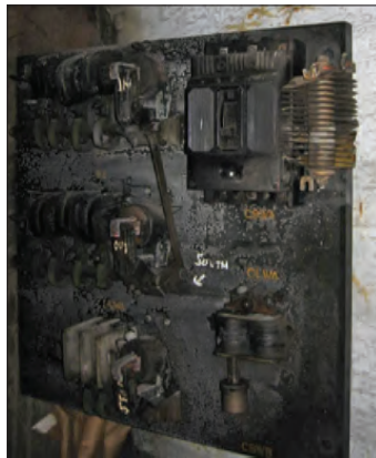
Circuit Breaker with Speed Control Winch
