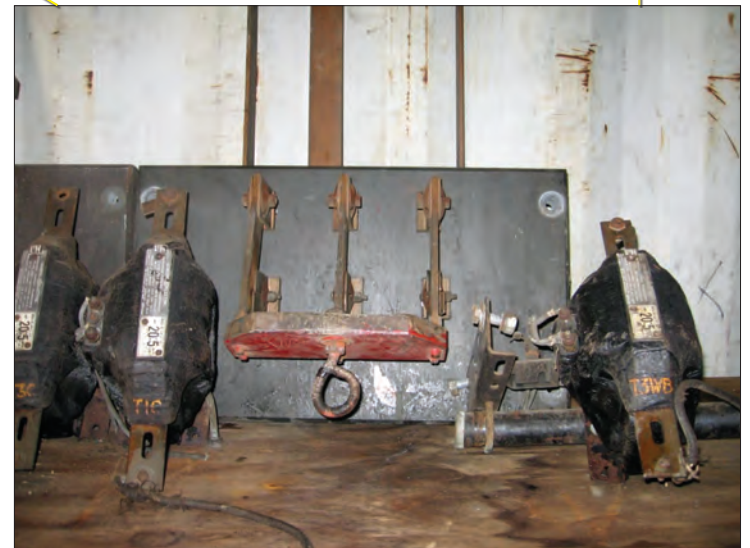
Phase Knife Switch and Transfers
